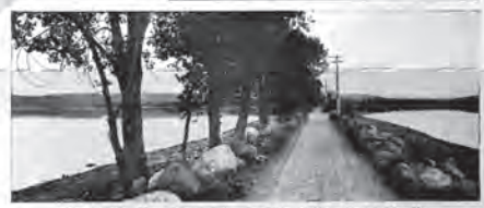
Part of the Hesse Island Trip—Sandbar Bridge, Grand Isle, Vt.
